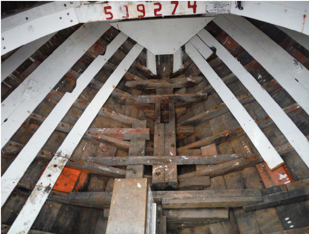
LOOKING FORWARD IN THE CABIN
