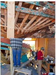
Work continues on schedule, with the first sheer planks fastened, spiling of the top transom plank, fitting of floor timbers and progress on the futtock replacement progressing through midship.
