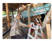
The full shipwright crew returned to the Woody on Oct. 11. Our volunteers worked to remove and fabricate the first seven frames port and starboard so that a portion of the crew would be able to work on
