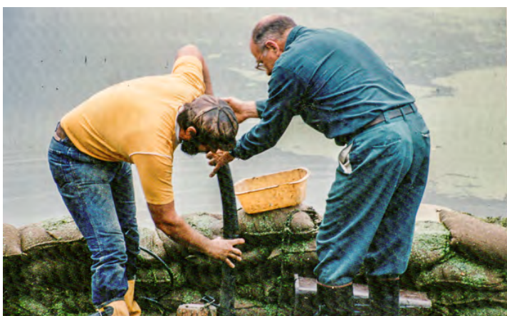
John Griffith during the building of the boat ramp Photo supplied by Mel Healy
